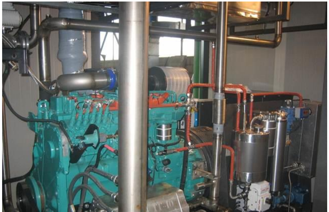
Inside the cabin of a 100 kW electric-thermal energy production generator designed by Powertron. The system works on an average of 650 hours/month continuously.
