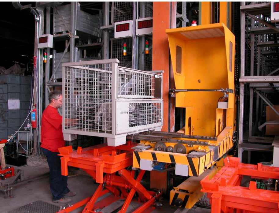
One of the loading/unloading bays. A weighing system makes an exact and precise calculation on goods available.
